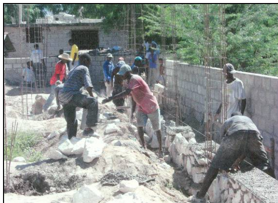
Figure 1 Nativity School Construction July, 2005
